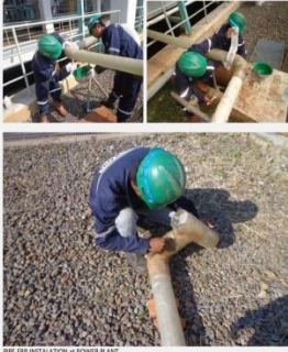
PIPE FIB INSTALLATION at POWER PLANT
