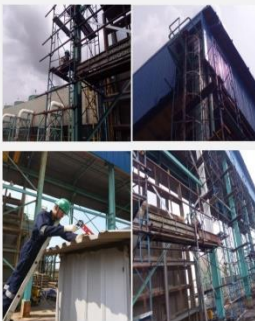
INSTALATION CLASING AND ROOF at POWER PLANT
