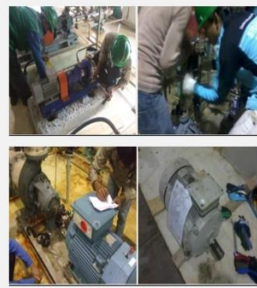
INSTALATION MOTOR AND ALIGNMENT at POWER PLANT
