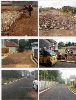
ASPHALT WORK at LAMPUNG RESIDENCE
