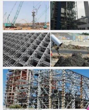
STEEL STRUCTURE WORK at POWER PLANT
