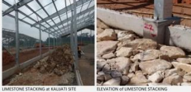
LIMESTONE STACKING at KALIATI SITE ELEVATION of LIMESTONE STACKING
